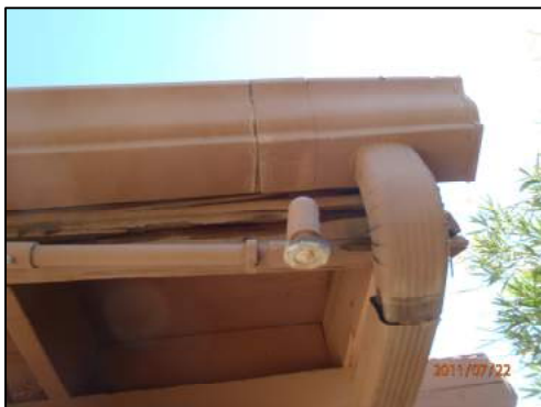
Left photo: Partially disconnected elbow at downspout.
