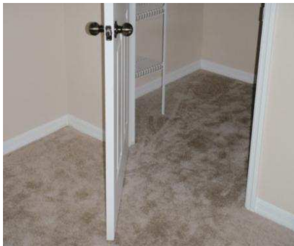
(Photo 2: Walls & Closet)
